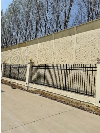
(PGTEX install sound insulation wall to control noise)
