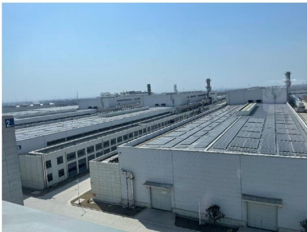
(PGTEX carbon fiber plant roof installation of photovoltaic)
